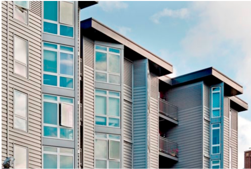
Matae Belltown Condominium in Seattle, WA
