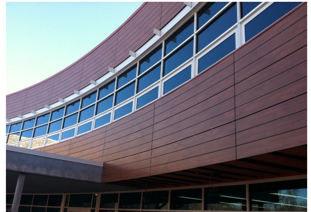
Orchard Place Elementary School - Des Plaines, IL Example of Face-scores on Trespa Panels emulating tongue and groove planks
