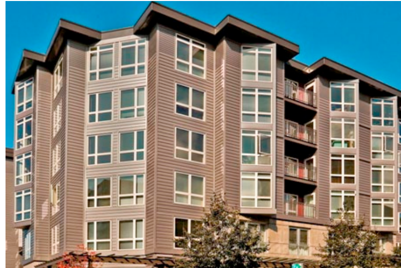
Matae Belltown Condominium in Seattle, WA
